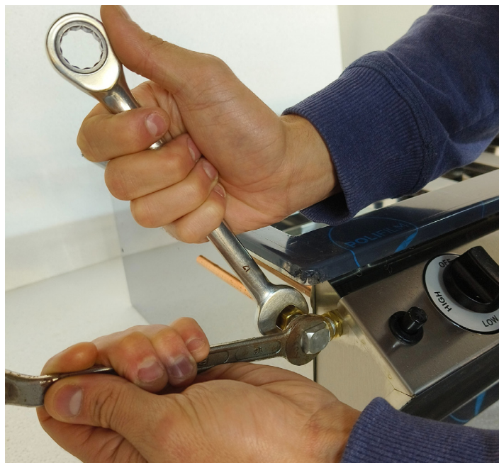
Fig 1: Connecting copper pipe to the aluminum elbow
